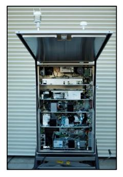
• Air Monitoring Trailer: The air monitoring trailer system will operate as a semi-mobile platform. This platform will be equipped with advanced air monitoring analyzers with the ability to communicate the community-level air quality in real time.
