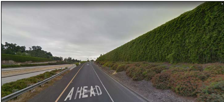
Figure 4-3 Vegetative Barrier w/ Solid Barrier on Highway 198, Visalia, CA
