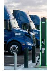
HD EV Charging Infrastructure
