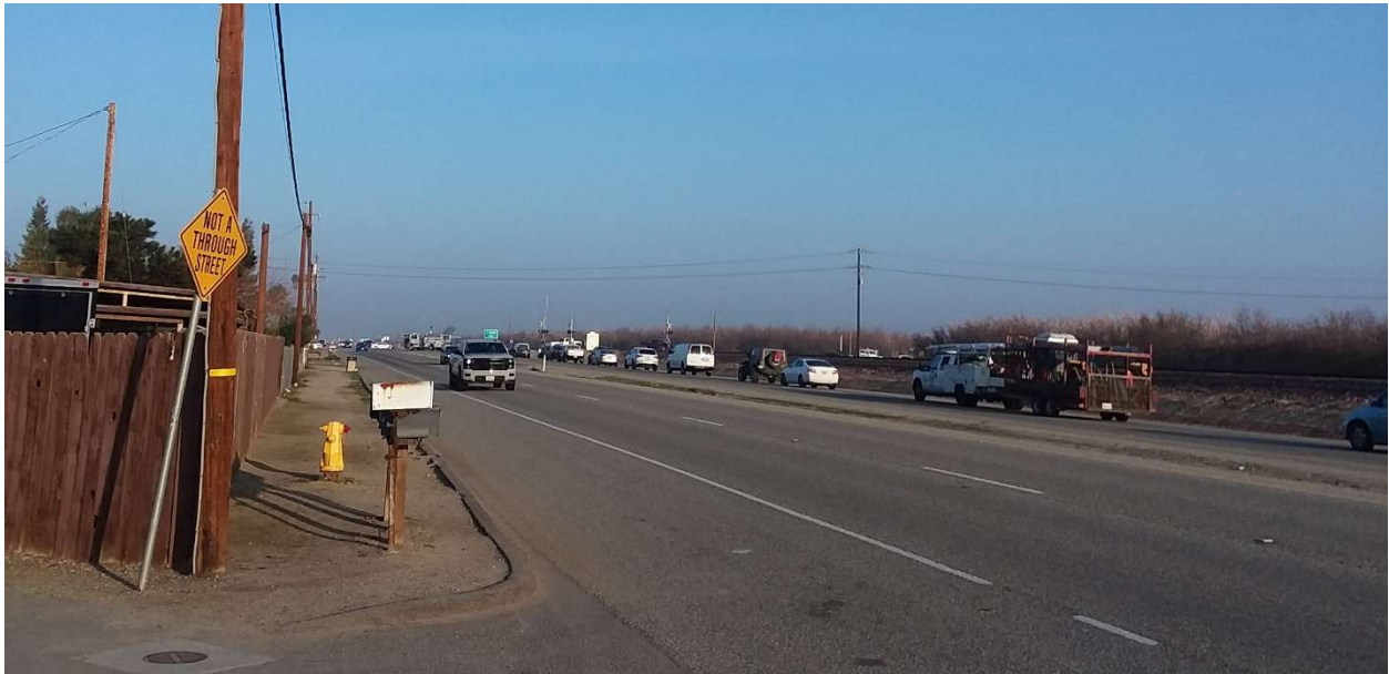
Figure 4 - Existing Highway 43 Shoulder Looking North
