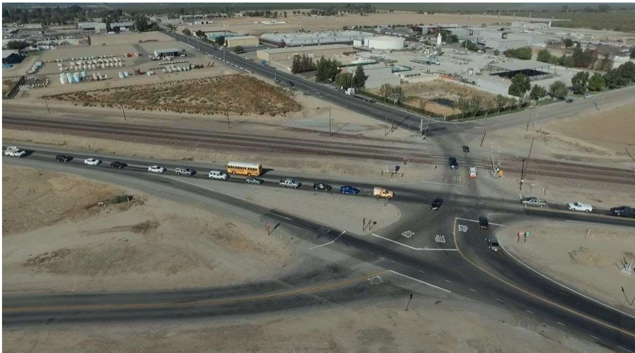
Figure 5 - Existing Roundabout Intersection
