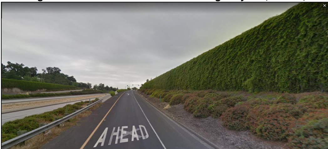
Figure 4-8: Vegetative Barrier w/ Solid Barrier on Highway 198, Visalia, CA*
